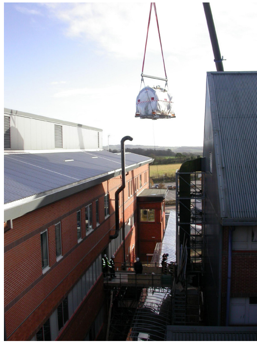
(Above) A sequence of images showing the delivery of a new MRI scanner which has to be craned into the building. The design of the hospital includes this gap between buildings to allow the crane to carefully lower the scanner. A removable wall allows the delivery and the heavy equipment can be moved directly into place.
