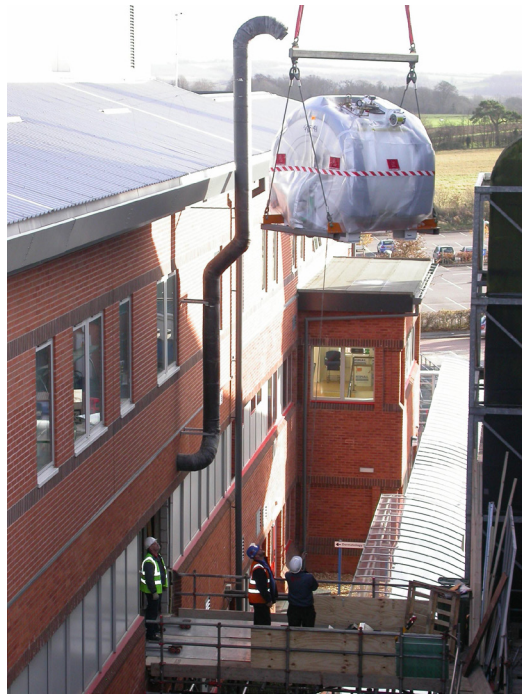
(Above) A sequence of images showing the delivery of a new MRI scanner which has to be craned into the building. The design of the hospital includes this gap between buildings to allow the crane to carefully lower the scanner. A removable wall allows the delivery and the heavy equipment can be moved directly into place.
