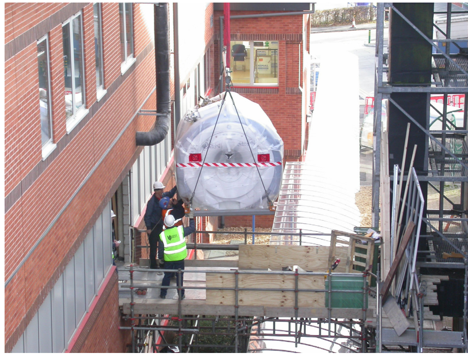
(Above) A sequence of images showing the delivery of a new MRI scanner which has to be craned into the building. The design of the hospital includes this gap between buildings to allow the crane to carefully lower the scanner. A removable wall allows the delivery and the heavy equipment can be moved directly into place.
