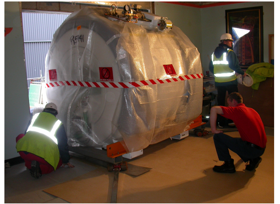
(Above) A sequence of images showing the delivery of a new MRI scanner which has to be craned into the building. The design of the hospital includes this gap between buildings to allow the crane to carefully lower the scanner. A removable wall allows the delivery and the heavy equipment can be moved directly into place.
